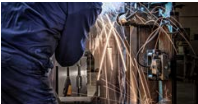
Welding of frame
